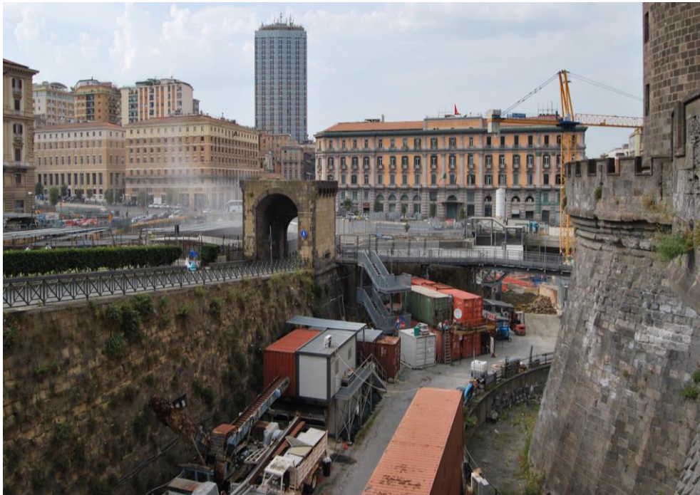
Fig. 4 – Metro’s works at Municipio Square, Naples, 2018
