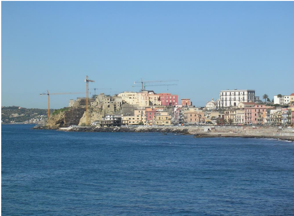
Fig. 16 - The Rione Terra from the sea during the restoration works
