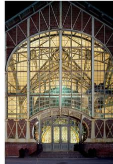
12. The Zollern 2/4 colliery's machine hall with the first electric hoisting machine at a main shaft was built as a steel framework structure with brick infill and decorated with Art Nouveau elements (Photo: LWL-Industriemuseen).
