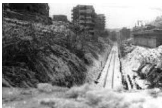
Pl. III.2 - View from the bridge over the Rome-Viterbo train tracks looking south. Source: Roma Sparita .
