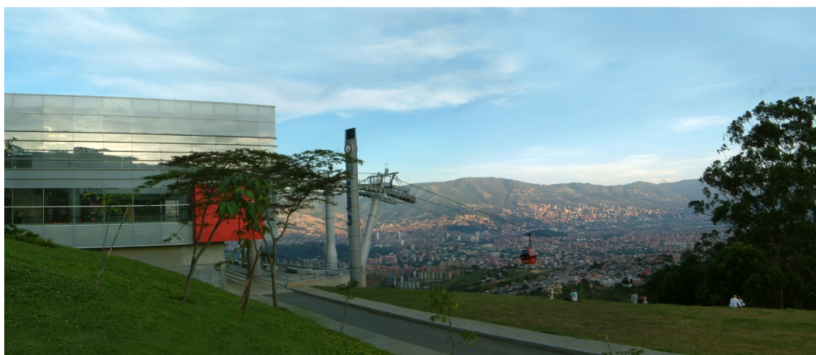
Fig. 9.- Terminal cable-car station of the West
