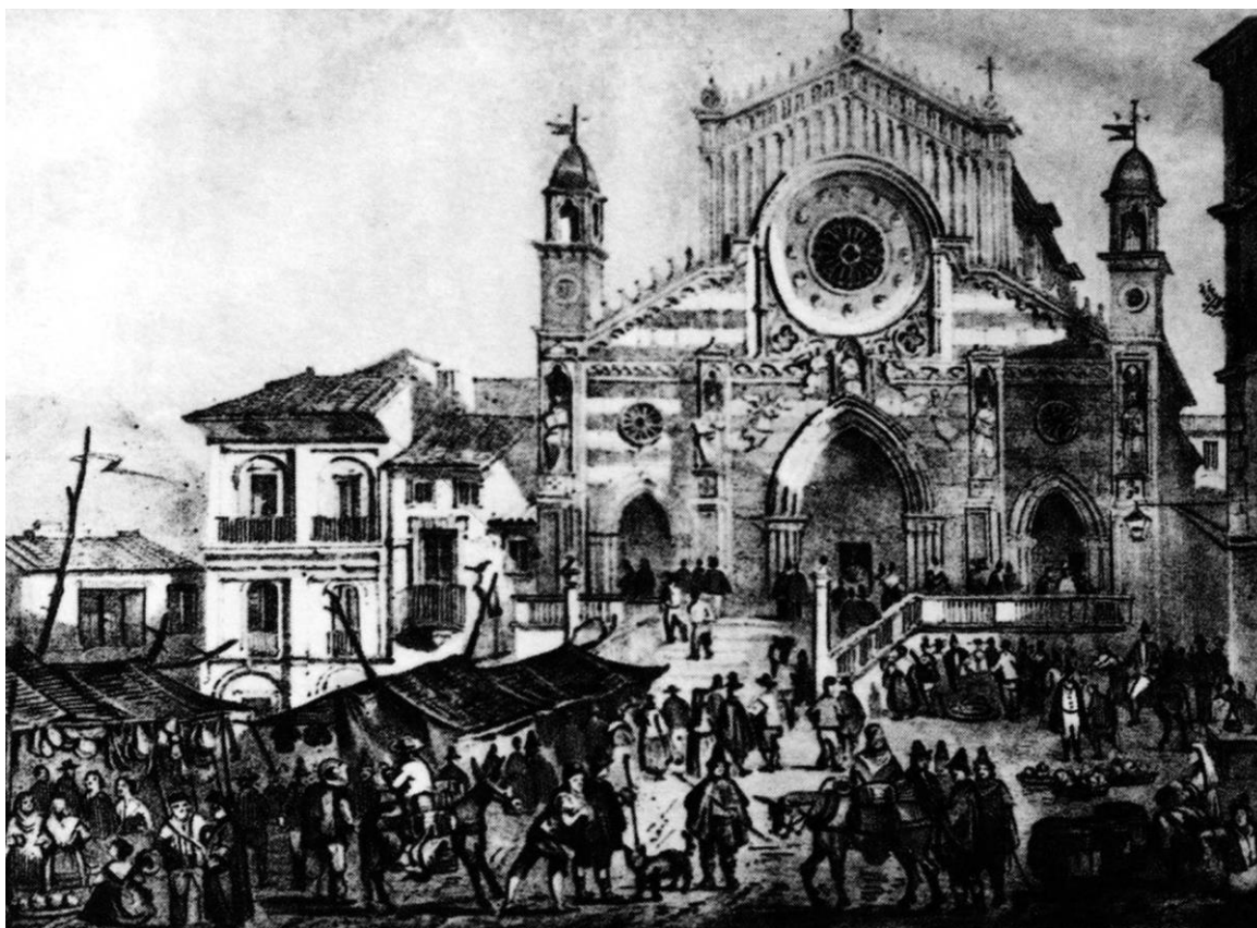
Fig. 2 The picture of the Cathedral's plaza of the eighteenth-century Cosenza
