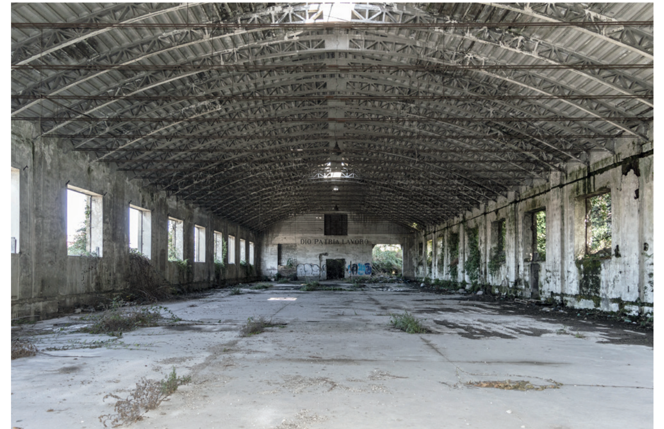
Figure 9: The inside of the first Kerasav warehouse: reinforced concrete trusses and fascist slogans. Source: own photo.
